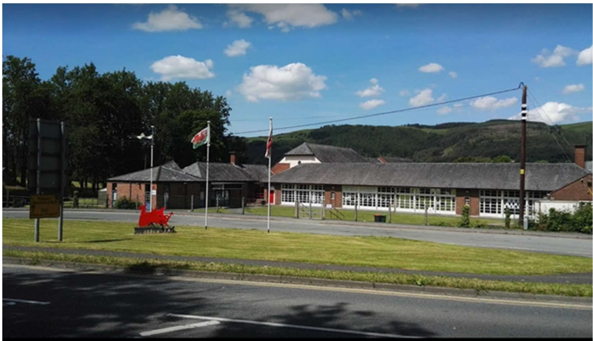
Figure 2: Secondary School Campus
